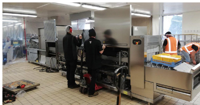
The new dishwasher being installed
