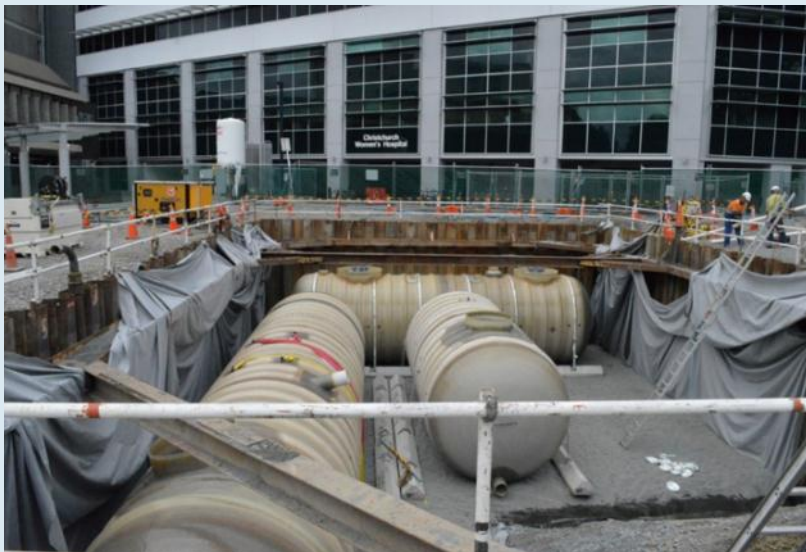
Above: Large tanks for diesel and sewage have been installed behind CWH.
