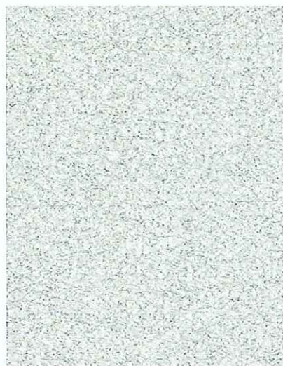
Fine through-colour finishing render on concrete blockwork Bedroom wing type 2
