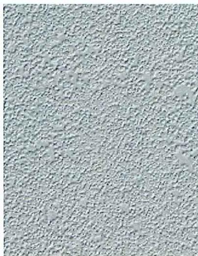
Rough (and brushed) through-colour finishing render on concrete blockwork Bedroom wing type 2 spandrel
