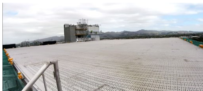
Orange PAL lights around the edge of the helipad
