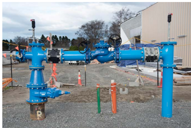
One of the wellheads the water will run through. The Energy Centre is in the background
