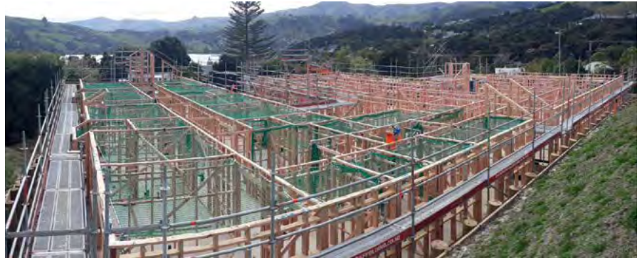
A panorama of the site shows the foundations in place and the timber framing for the walls going up.
