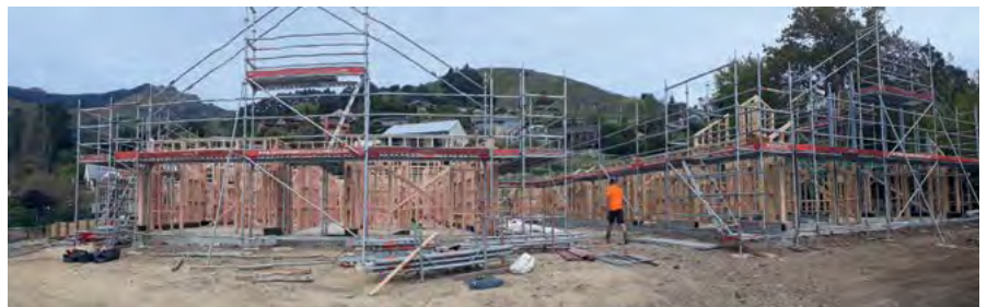
Scaffolding going up around the site for the timber framing that will form the two gables.
