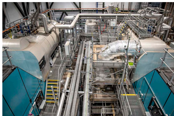
Looking down on the two silver biomass boilers and teal combustion chamber
