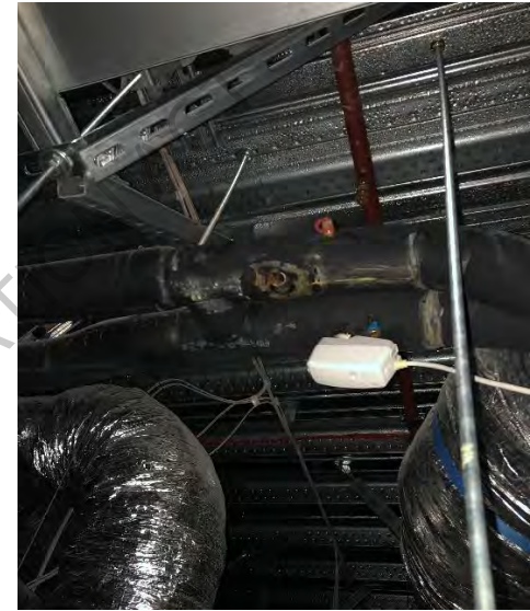
Image 4 – Drain valve location
