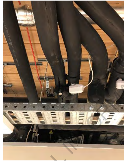
Image 3 – Drain valve example location
