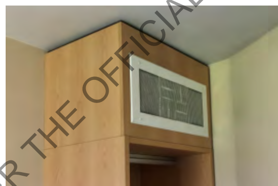
Supply air diffuser in bedroom incorporated into bedroom wardrobe.
