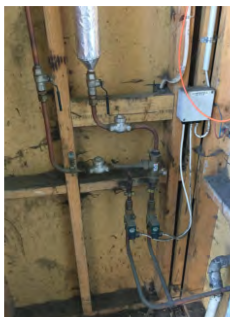
Pipework insulation has been provided on the hot water pipework, however both the hot and cold water pipes should be insulated as they are located in an uninsulated service cupboard.
