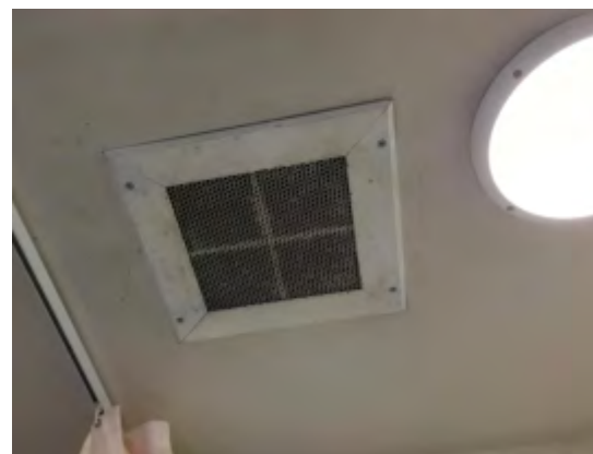
Supply air diffuser in bedroom incorporated into bedroom wardrobe.
