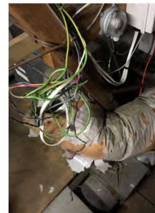
Further examples for the poor ductwork condition is evident in the photos above, also visible are modifications to the control wiring which has been modified and or replaced in an untidy manor with the redundant cabling being left in place.
