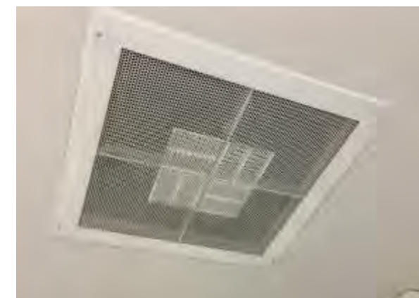
Ceiling air diffusers in bedroom, in 'Te Whare Hohou', neither building have used anti-ligature ceiling diffusers.
