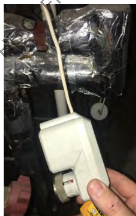
Pictured above is a 3 port valve motorised valve actuator which should be controlling the output of the FCU heating coil. This valve acutator has been detached and left sitting next to the unit, this eliminates the control ability of the FCU.
