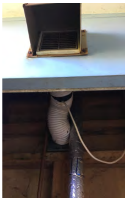
Pictured above is a defective bathroom fan from one from bedroom G058. If these systems are not operational they should be removed.
