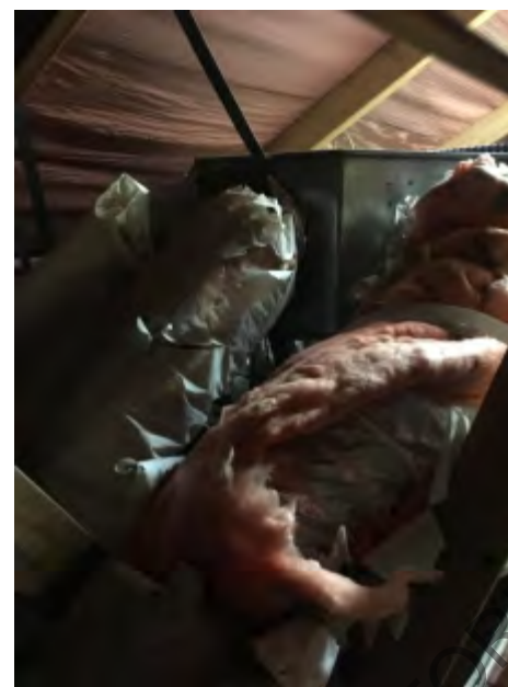
Shown in the photos above is the condition of the fan coil unit secondary ductwork, the efficiency of the system will be greatly reduced due to its poor condition. Design airflow will also be greatly reduced due to the pinhole leaks etc. in the ductwork network.
