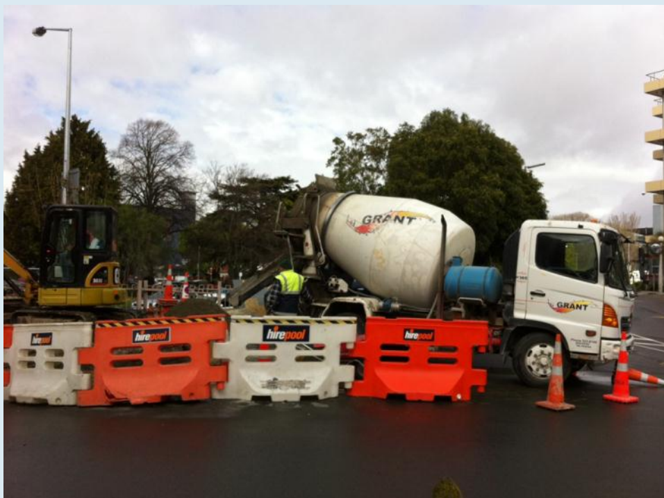
Above: The first (small) concrete pour on site at Christchurch!
