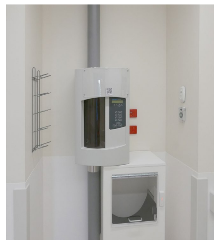
One of the 21 tube stations around the building. The system is a new version of what is already in use in other Canterbury DHB facilities so staff will be familiar with how it works, but will receive training during building orientation in October
