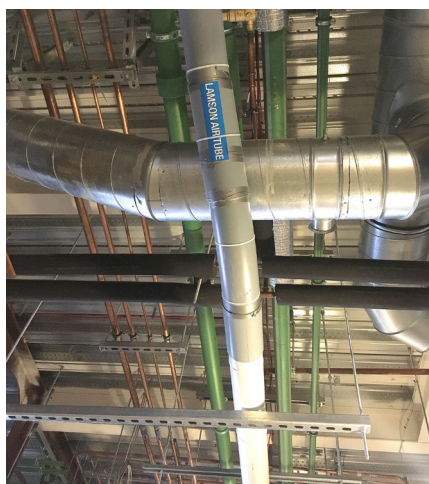
An example of the kilometres of pneumatic tubing that stretches through the ceiling spaces of the Hagley building
