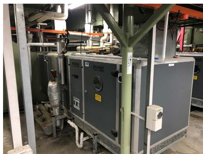
A typical air handling unit for an operating theatre in the Parkside plantroom
