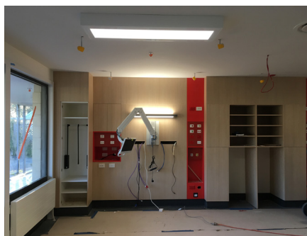
Test fit of the bracket and arm for a patient television. This will allow a patient to view the television from any position when they are in bed
