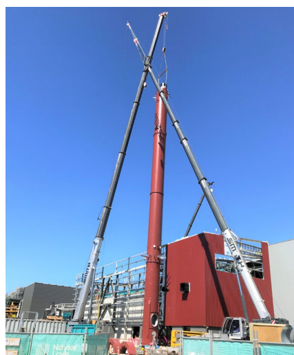
The last piece of the new chimney being attached
