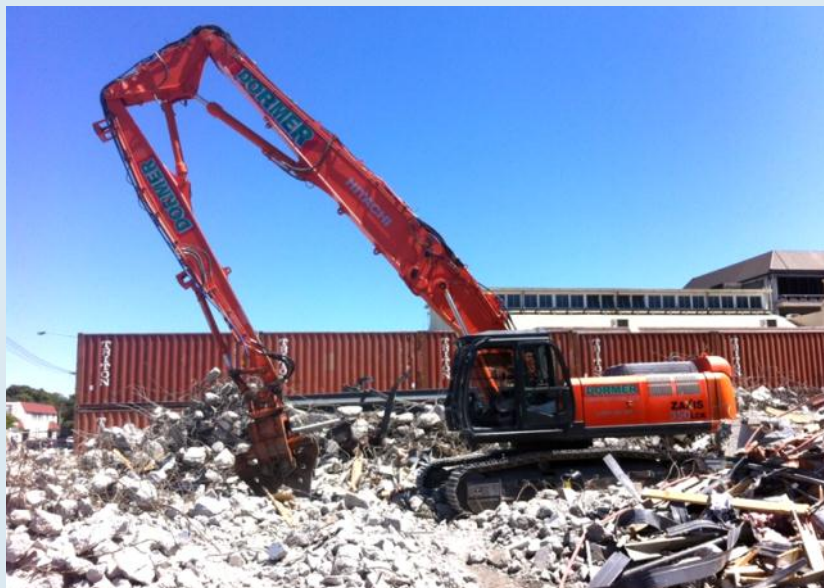
Left: A crackerjaw has made short work of the building at 41 St Asaph Street.
