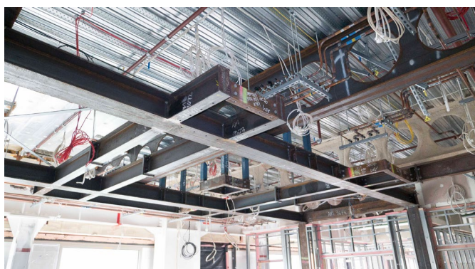
Secondary steel framework designed to hold the weight of the equipment
