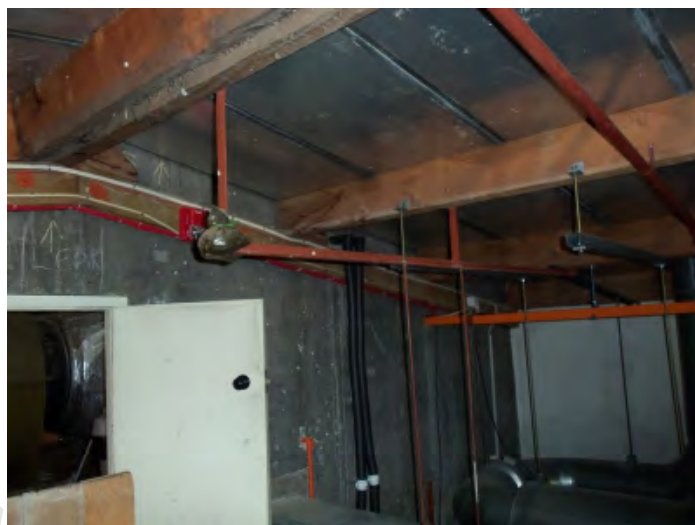
Figure 2-3: Roof Structure – “Woodtex” Panels on Timber Purlins
