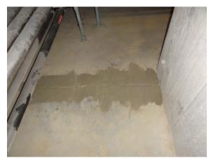
Figure 3-1: Evidence of Liquefaction below slab in service tunnel
