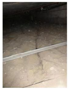
Figure 3-1: Evidence of Ground Fissures and Liquefaction
