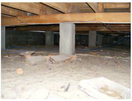
Figure 2-10: Internal Pier (Vertical Bolt Through)
