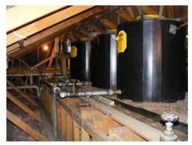
Figure 2-11: Water Tanks in Roof Space (Braced in Both Directions)
