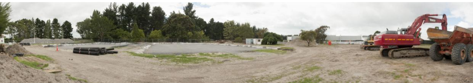
Above: Work is underway at Burwood Hospital.
