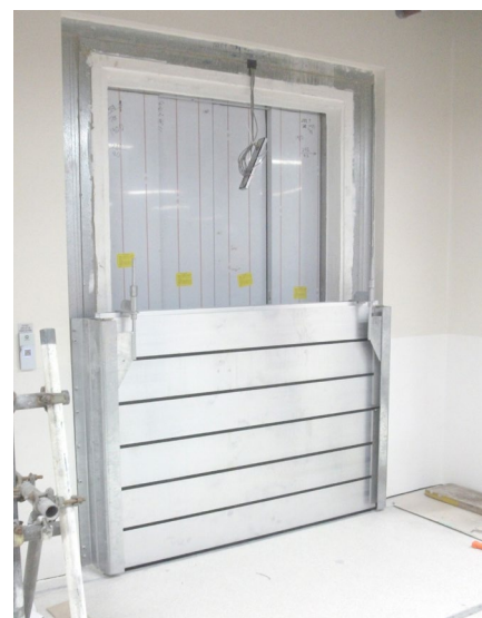
The lift with the barriers in place
