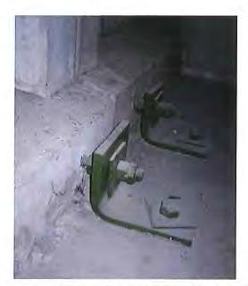
Figure 2-15: Bottom Precast Panel Connection - Block D Plant Room Level
