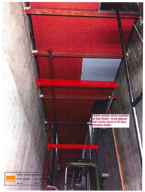
Figure 29: Access through Service Duct - underside of Level  $\bf 6$  showing proposed strengthening at floor levels
