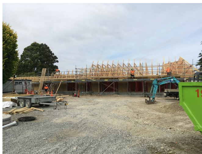
Eastern view of the extension showing the roof trusses going up
