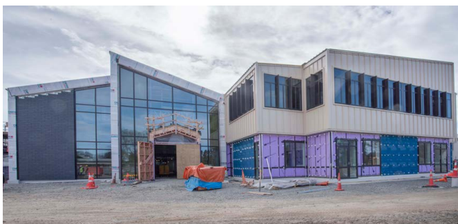
The exterior of building 14
