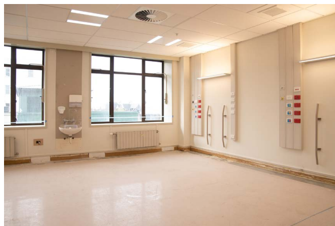
The refurbished four-bed room with new medical service panels
