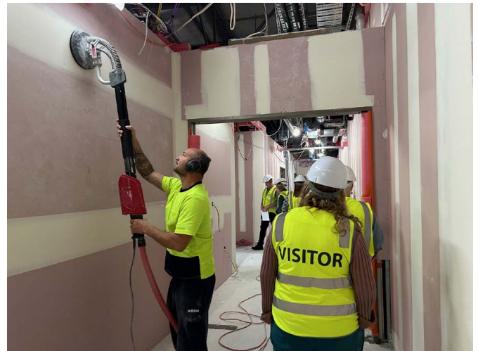
Work underway on the interior of Kurawaka Waipapa
