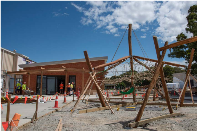
Playground under construction
