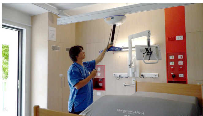
A ceiling hoist in a patient's room makes all the difference for patients and staff
