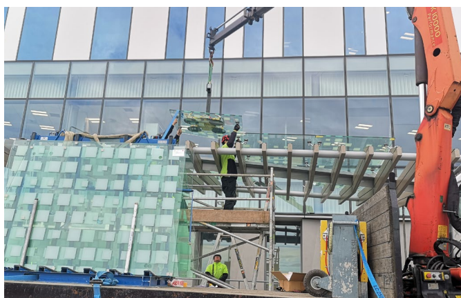
Glass being installed on the Super Stop on the north side of Tuam Street
