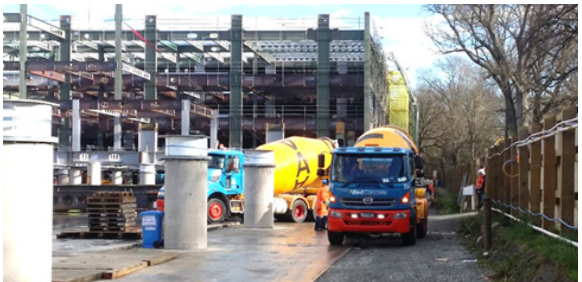
The photo to the right shows trucks in position at ground level to deliver the concrete – 195 cubic metres were poured in total.
