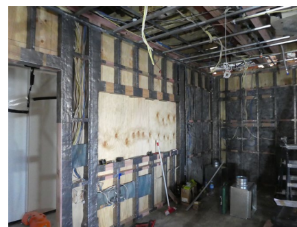
Lead walls being installed
