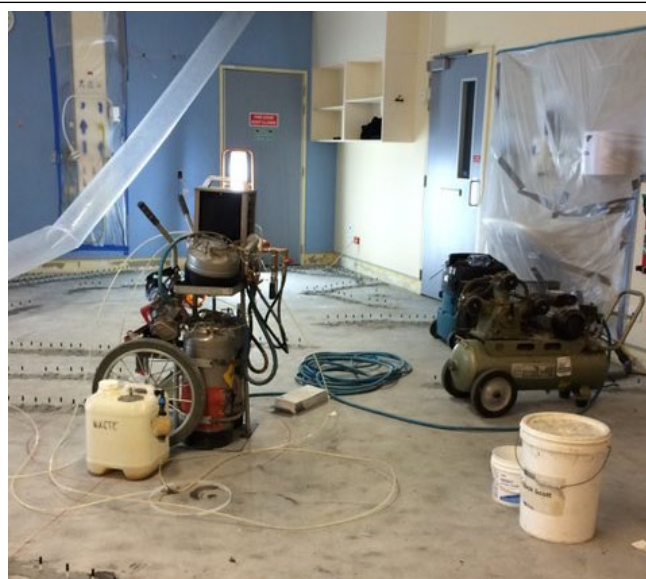
Above: Resin-injecting cracks in the floor of NICU.
