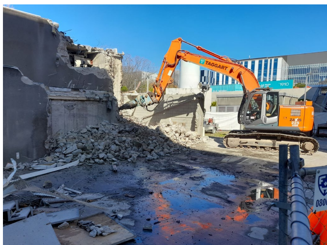
Hydraulic multi-processor unit being used to crush the existing generator building concrete roof and walls
