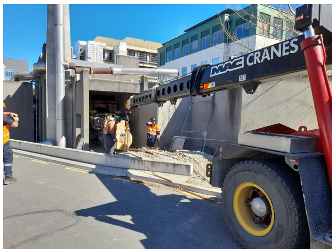
The original generator being removed before the demolition of the generator building superstructure
