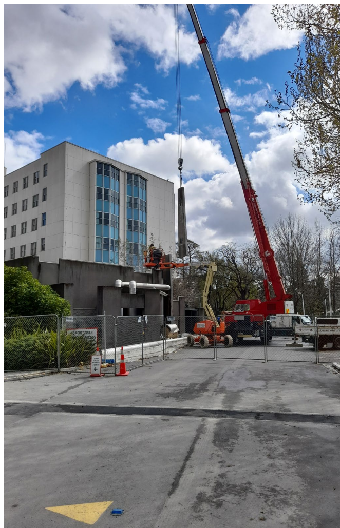
The top section of the concrete panel that supported the twin flues of the generator building being removed
