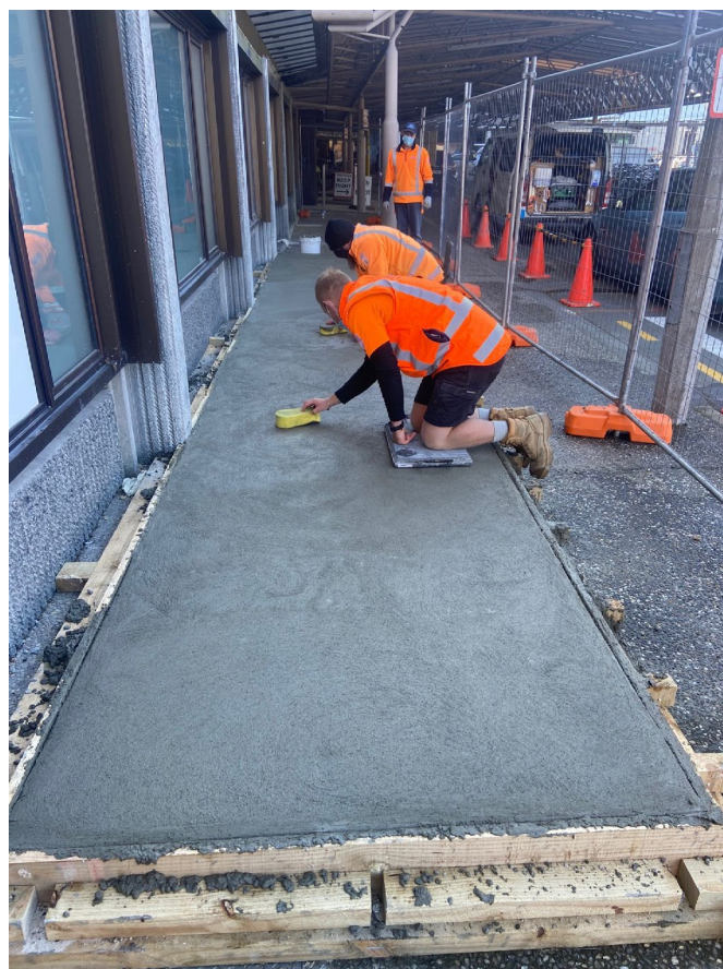
New concrete bases being prepared. Two large fans will sit on these bases as part of the ventilation upgrade for the ward
