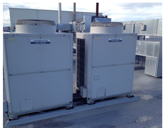
Above: Two large outdoor air conditioning units that produce the primary heating and cooling to be used by the indoor units.
