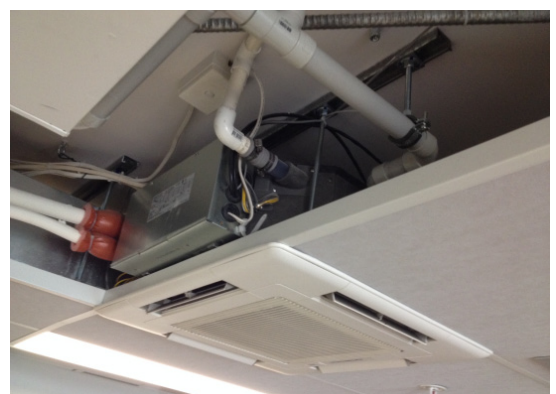
Above: The ceiling cassette units that provide individual heating or cooling at the Rangiora Health Hub.
