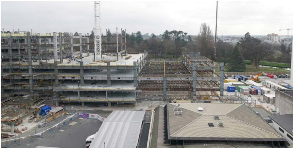
This wide angle shot of the ASB shows the west tower (on the left) with the steel framing up to level 6, the central core that stays at 3 storeys and the framing on the east tower with preparations underway for the first of several concrete pours that will form the floors of the tower.
