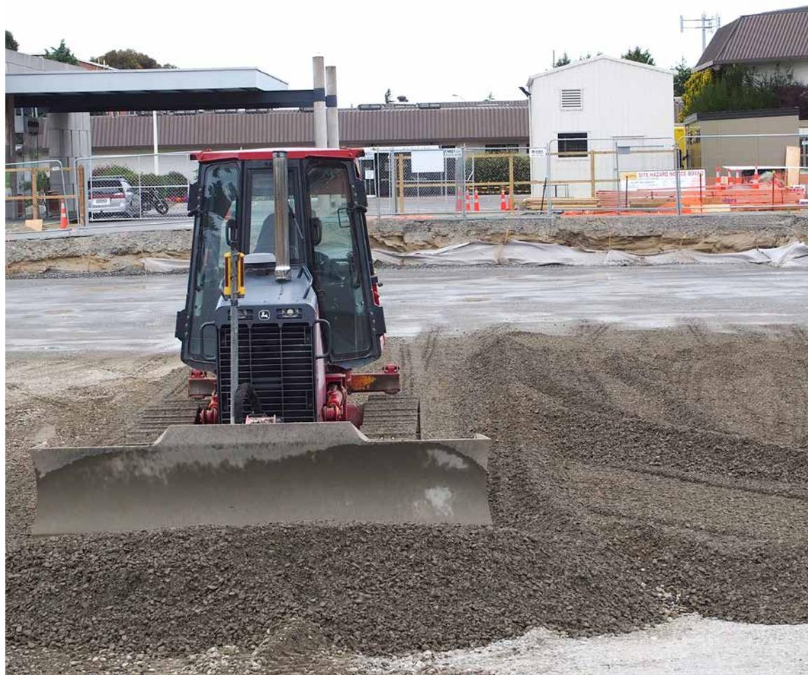
*Graders work on preparing the hardfill base ahead of construction starting on the new Burwood back of house.*
